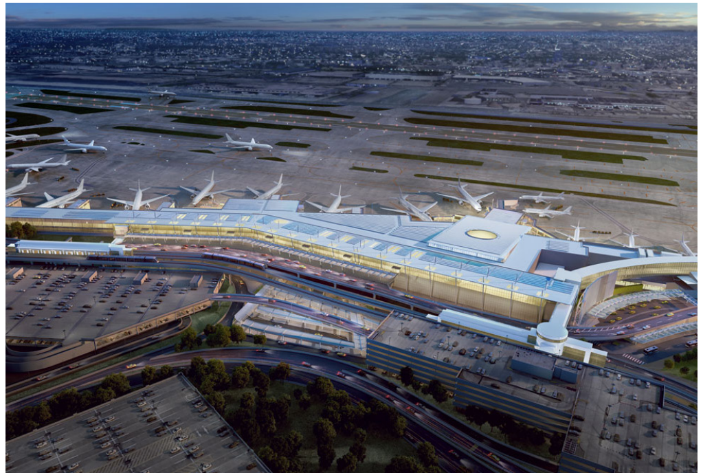
Rendering Courtesy of the Port Authority of New York and New Jersey
