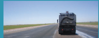
RUNWAY RUBBER REMOVAL
