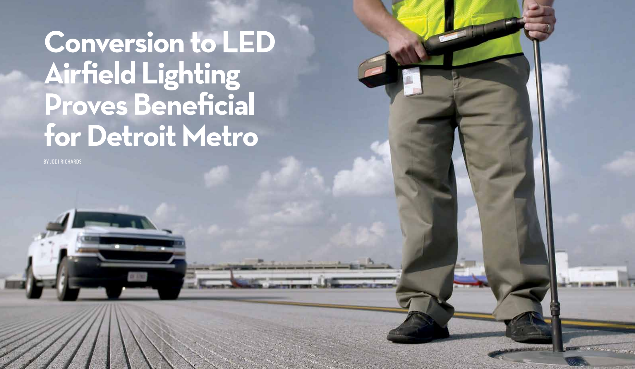
Data about torquing of in-pavement lights is transmitted via Wi-Fi for tracking and analysis.
