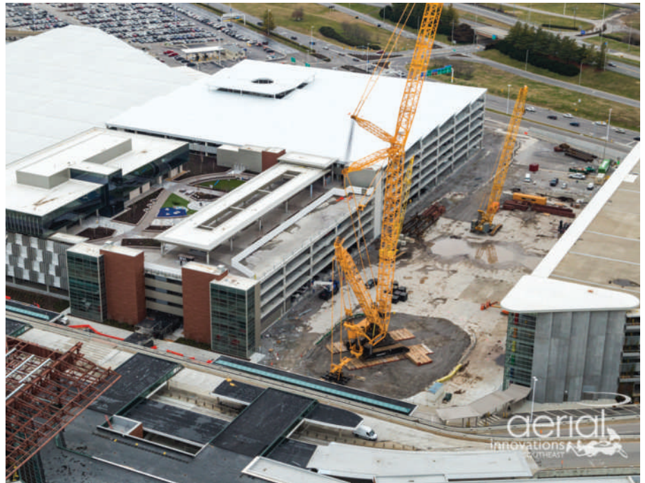
The new six-story garage was built in 18 months and opened in two stages.
