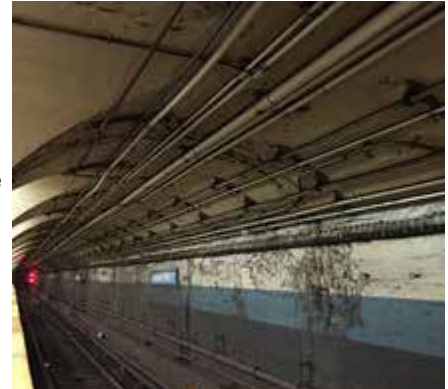
Existing Station Condition
