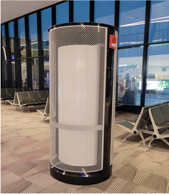
A custom displacement ventilation system helps control temperatures in passenger areas while reducing energy consumption.
