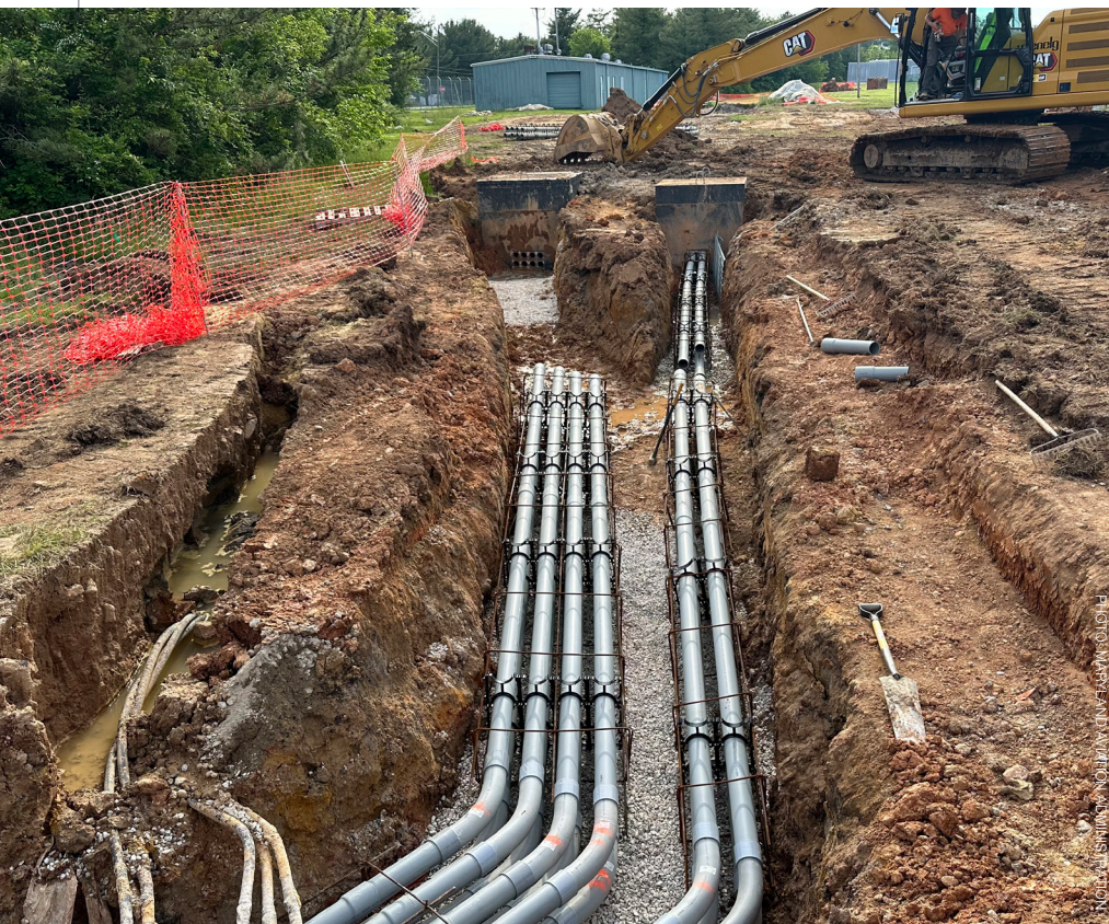
Installing duct banks before nightly runway closures began gave contractors a head start on the project.
